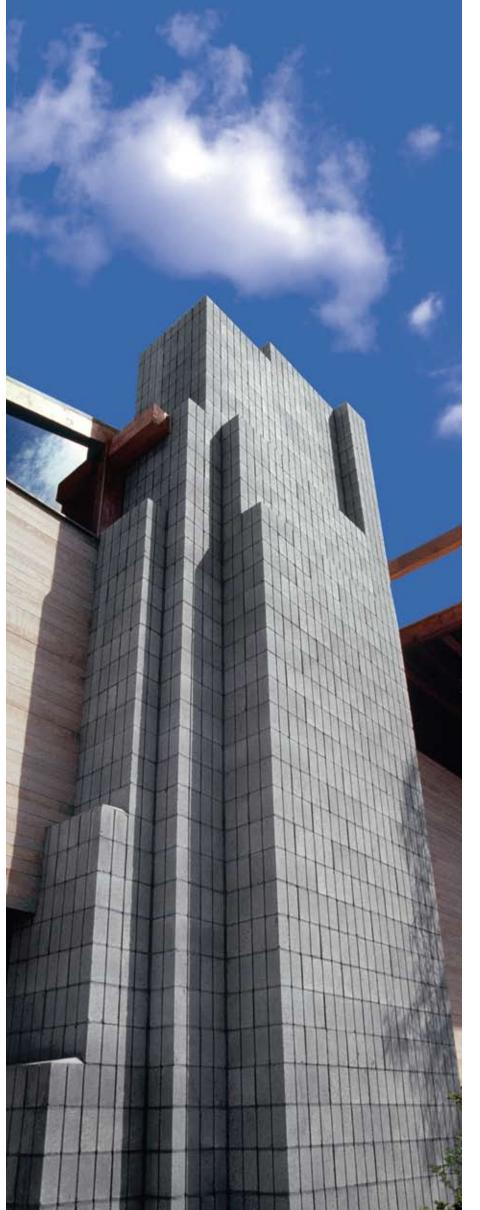
LEFT: What appears to be a skyscraper is really a chimney that scales one side of the home rising up 25 feet. An Applebaum innovation, exposed concrete blocks stacked with reinforced steel allow the structure to cantilever back into the chimney mass for seismic stability of the architecture.
